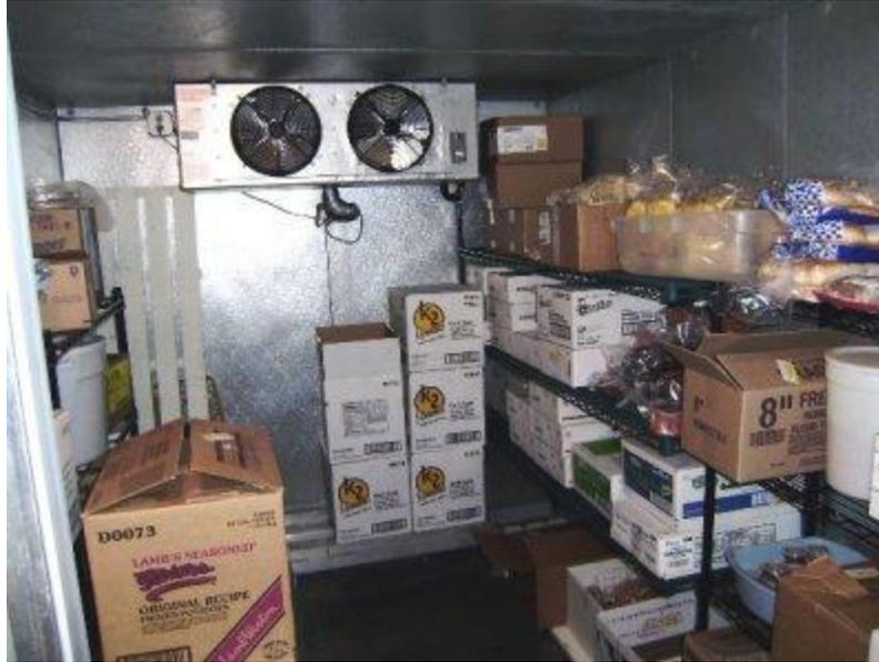
Figure 3: Walk-in refrigerator interior showing challenges to uniform airflow from chiller fans.
