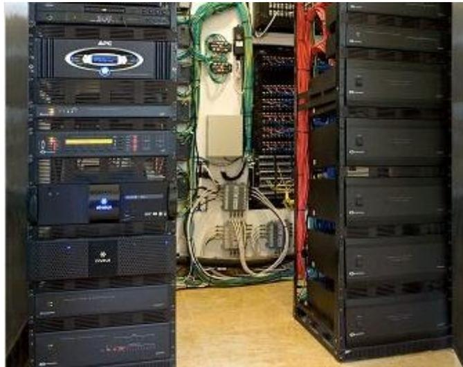
Figure 2: Server rooms present challenges with floor to ceiling and rack temperature gradients.
